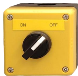
Figure 19 The image of accident ventilation start/stop switch
